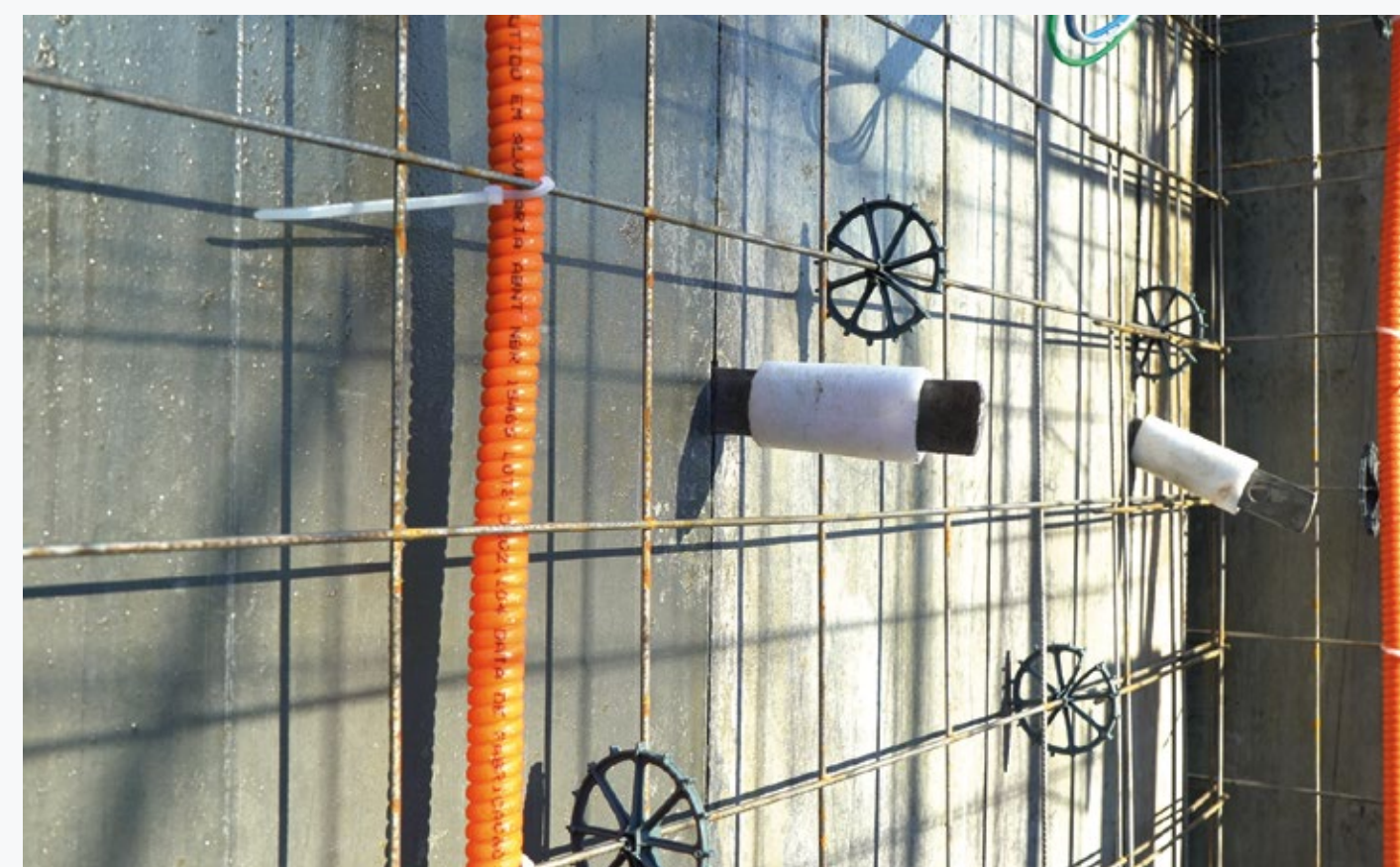
Camisas protegendo as sapatas
